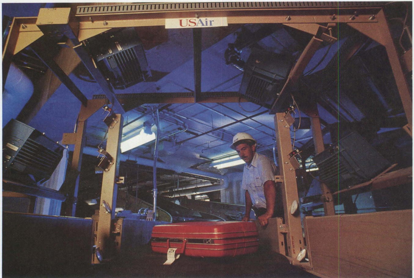
USAir's State-of-the-Art Baggage Handling System
